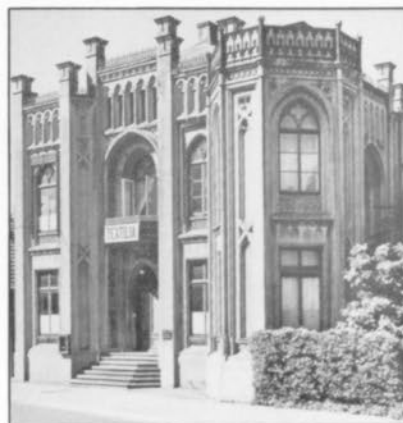
Neue Straße Nr. 16 in Weener
